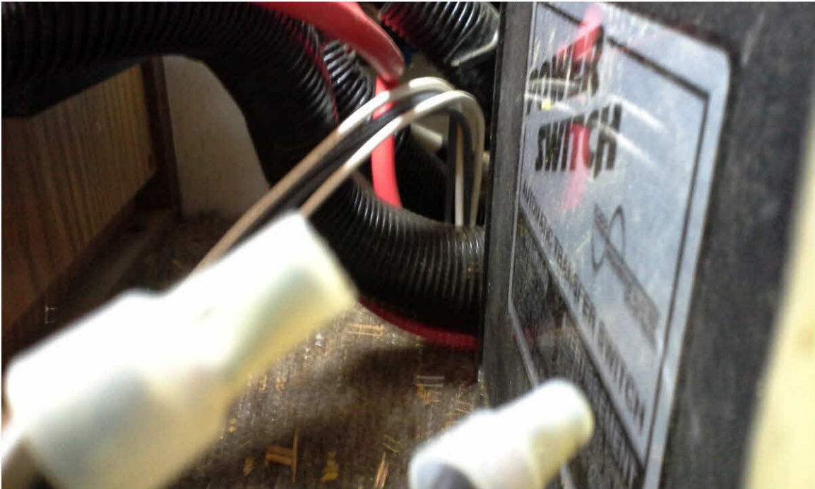
Looking in through hole where propane detector was removed
